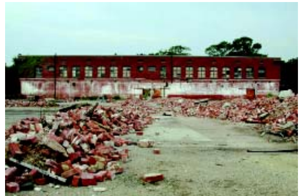
Rear of Administration Building
