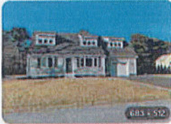
Past Projects - Falmouth Housing Trust falmouthhousingtrust.org
