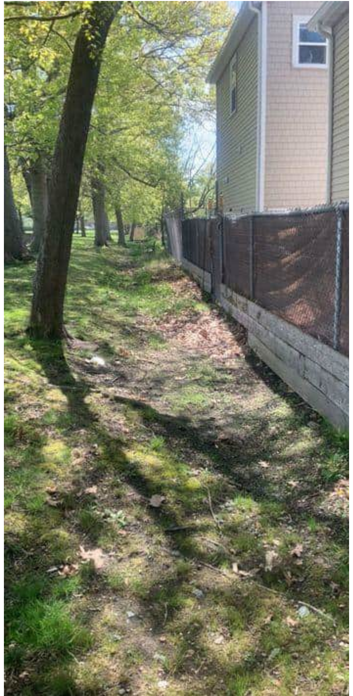
Section of swale leading to infiltration basin
