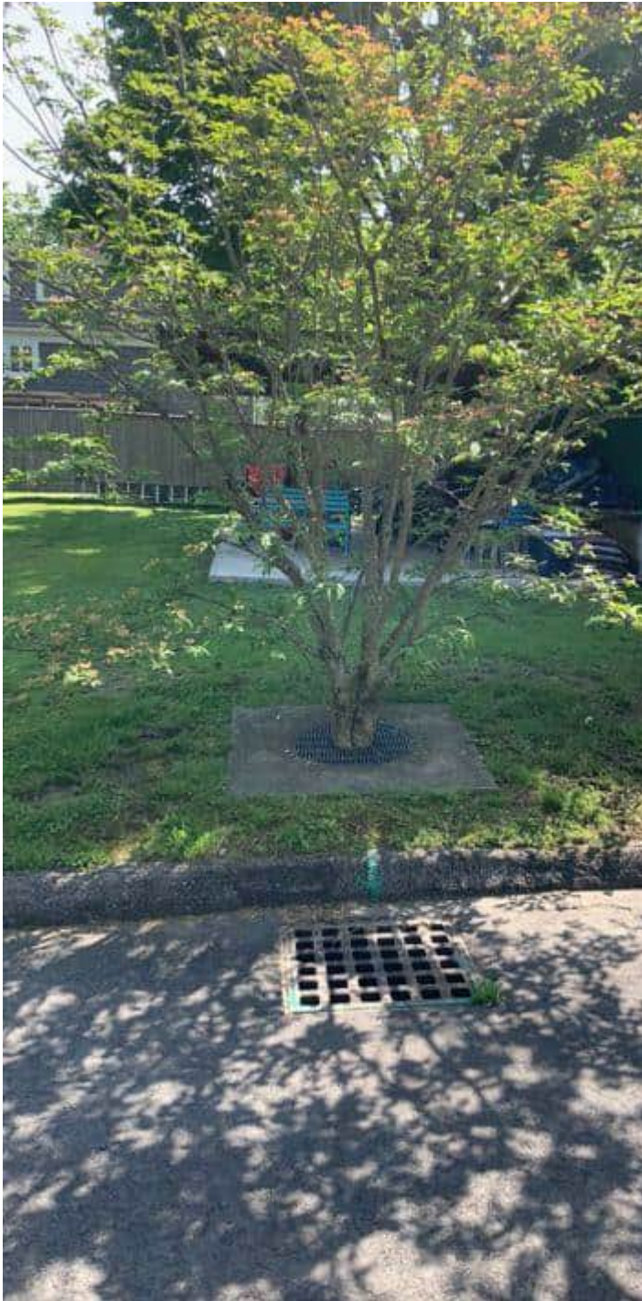
Outside tree box filter 1
