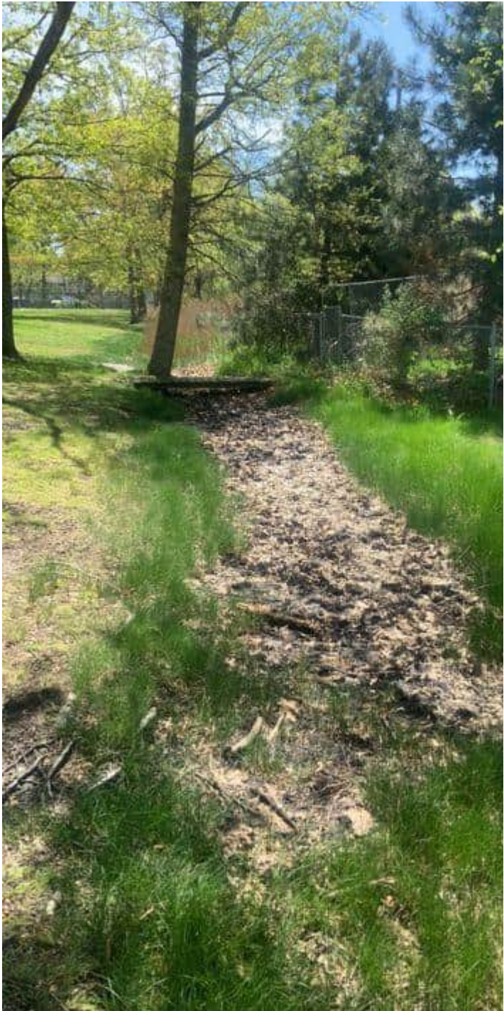
Section of swale leading to infiltration basin
