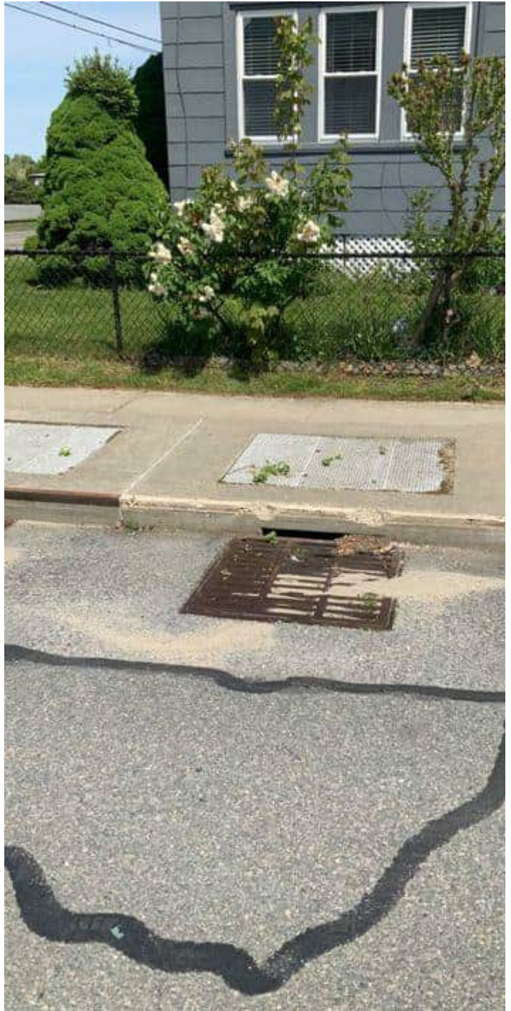
Inside tree box filter 2
