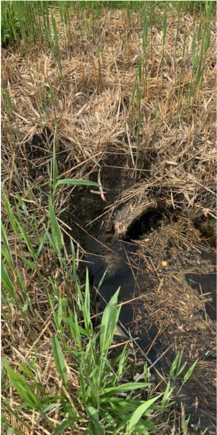
Swale inlet from CB
