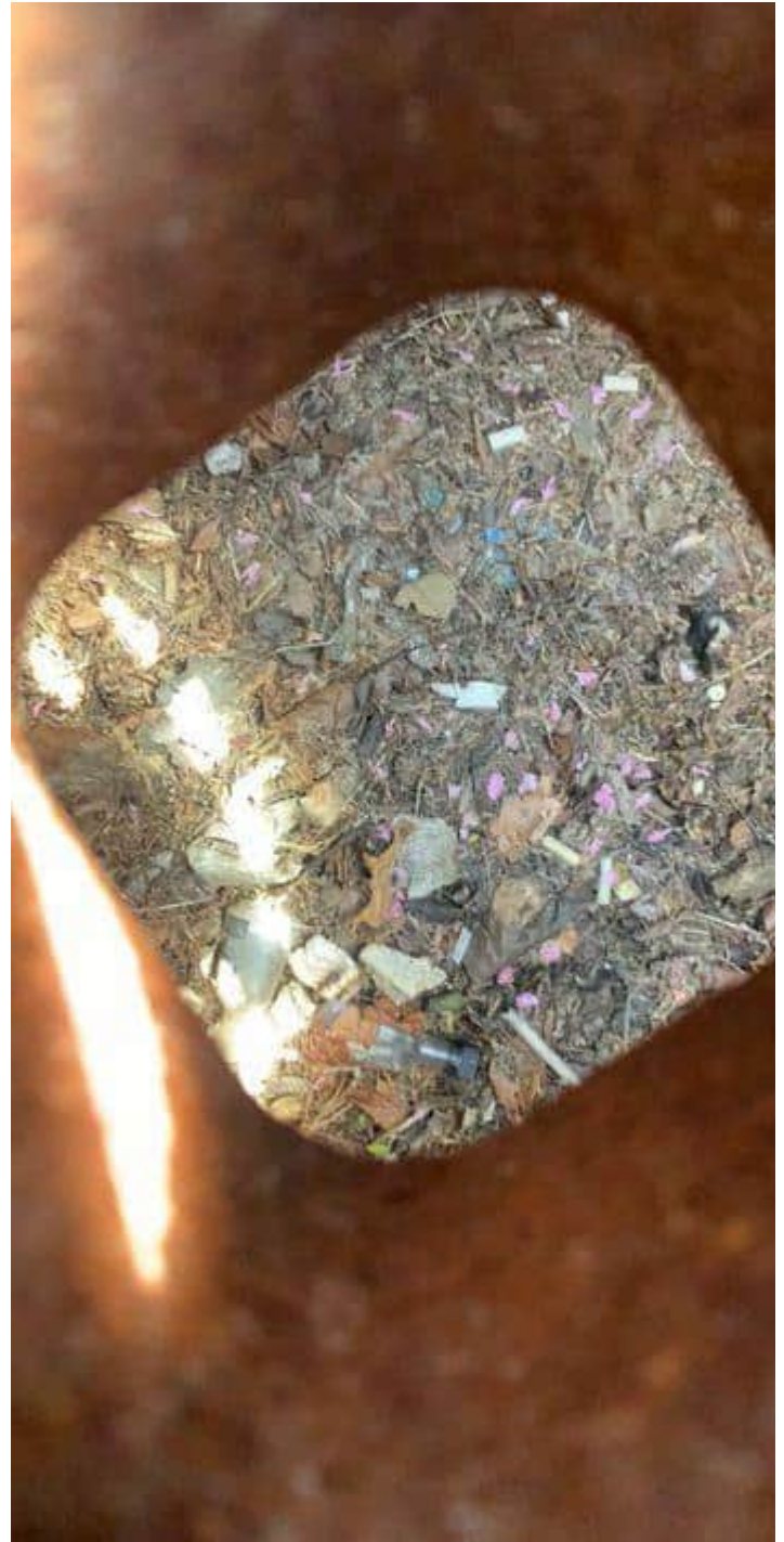
Inside tree box filter
