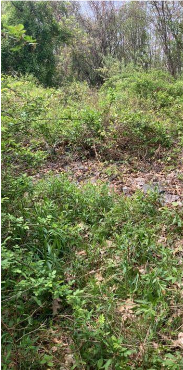
Basin outlet emergency spillway
