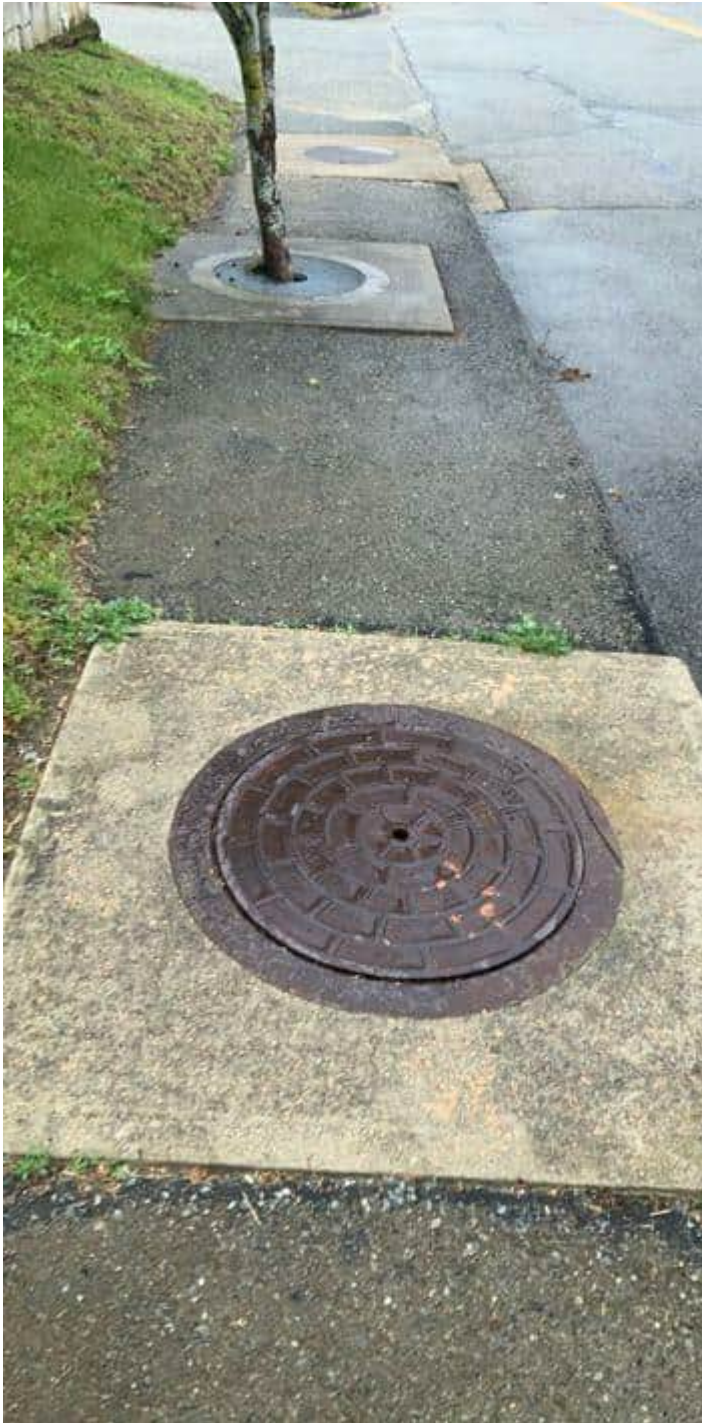
Outside pretreatment sump
