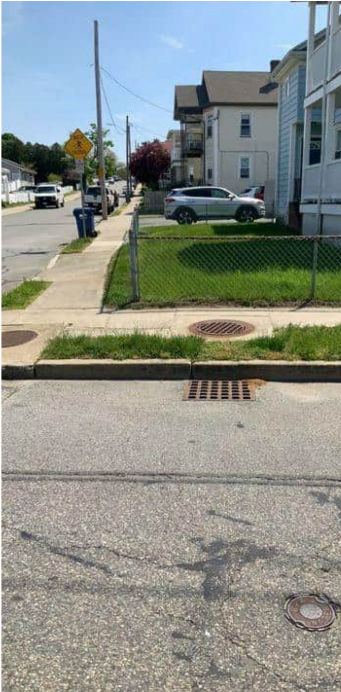
Outside tree box filter
