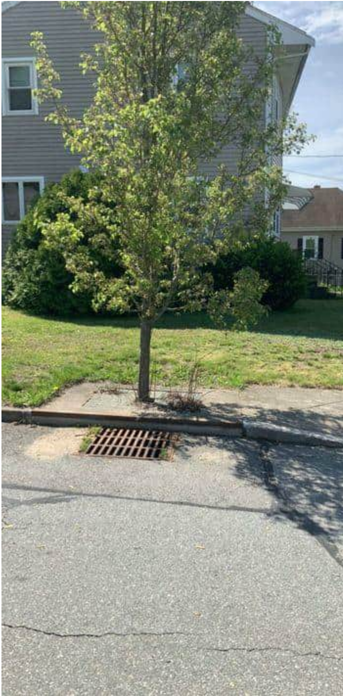
Outside tree box filter 1
