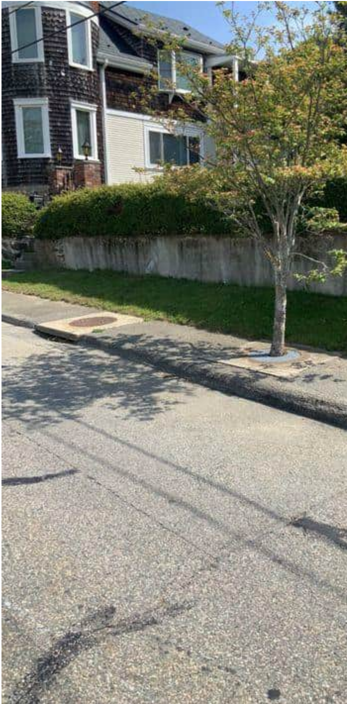
Outside tree box filter
