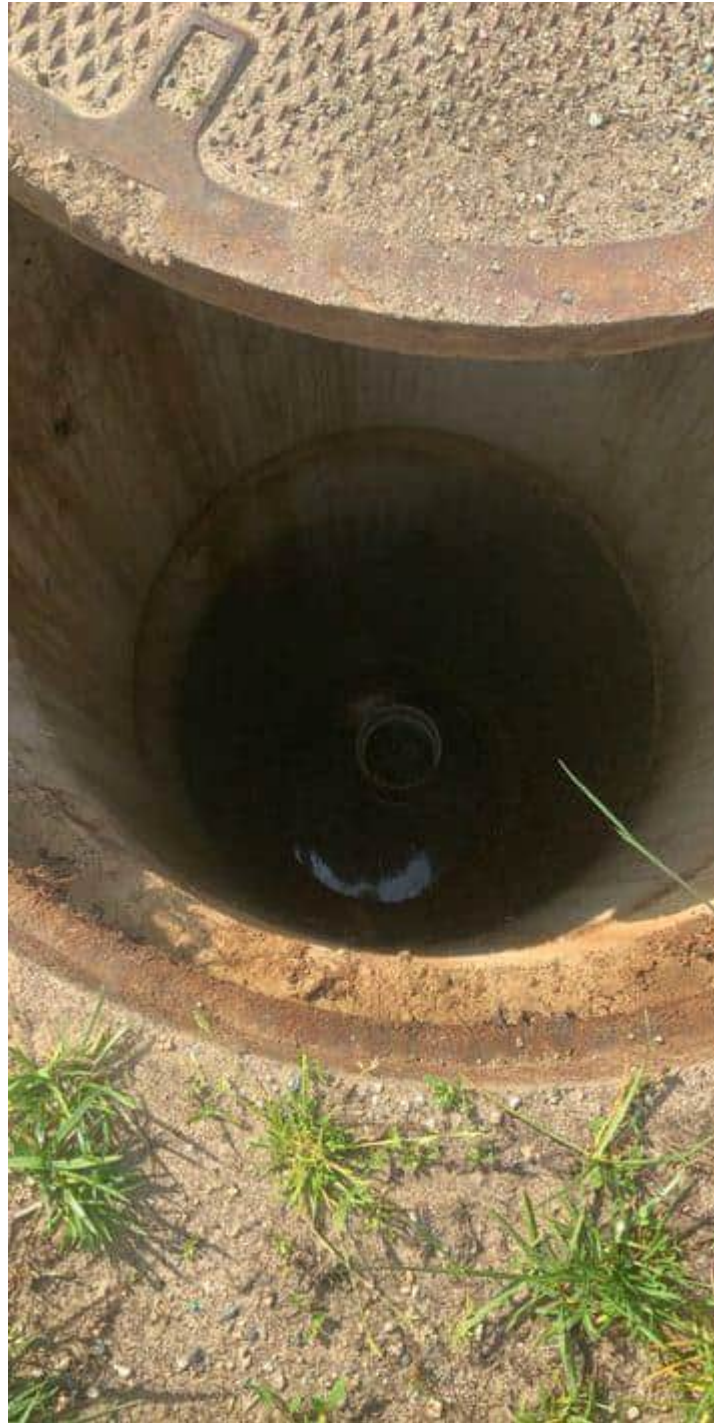
Inside outlet manhole
