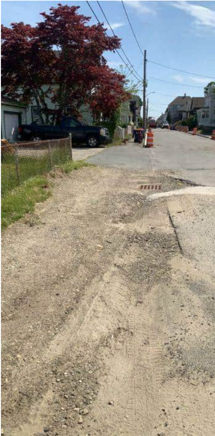
Outside tree box filter 2 removed under construction
