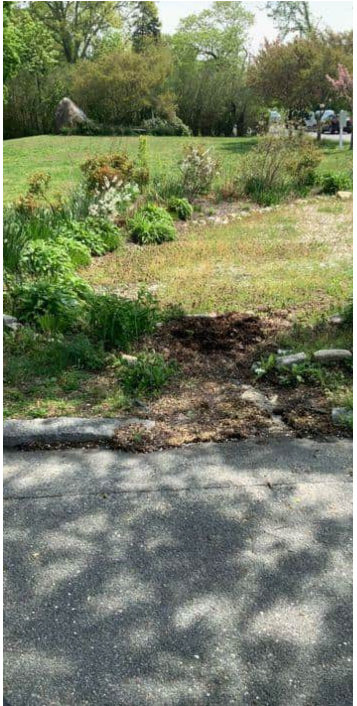
Rain garden inlet
