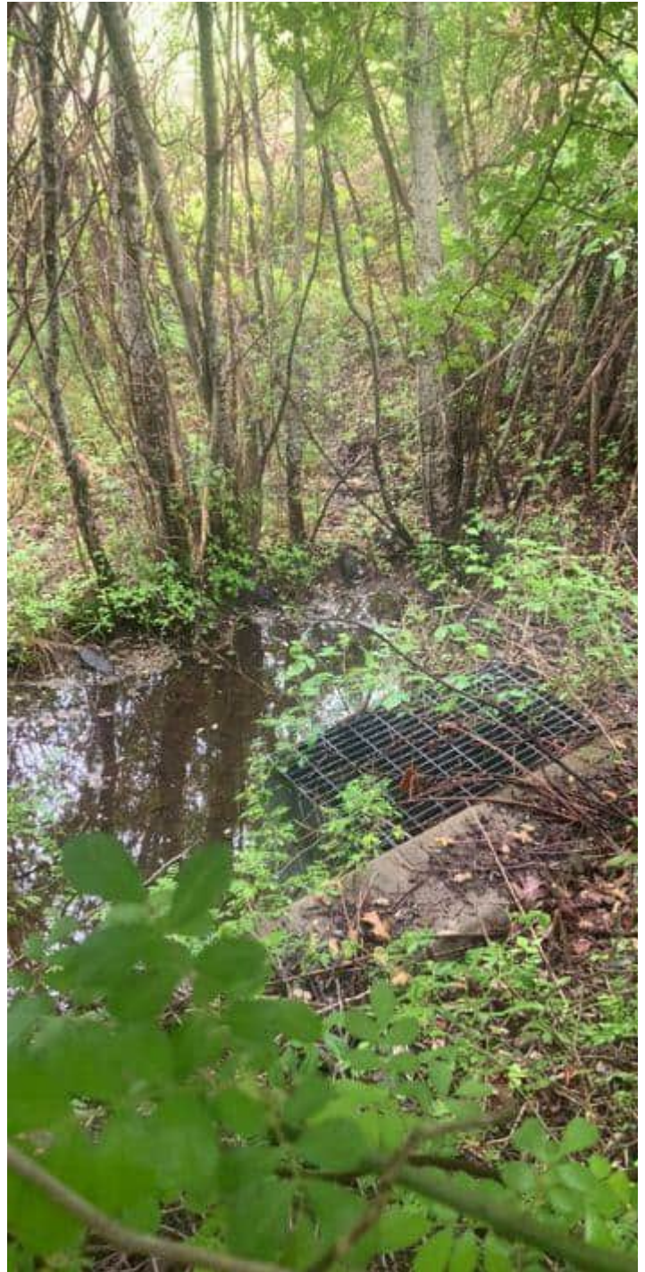
Basin Outfall Structure
