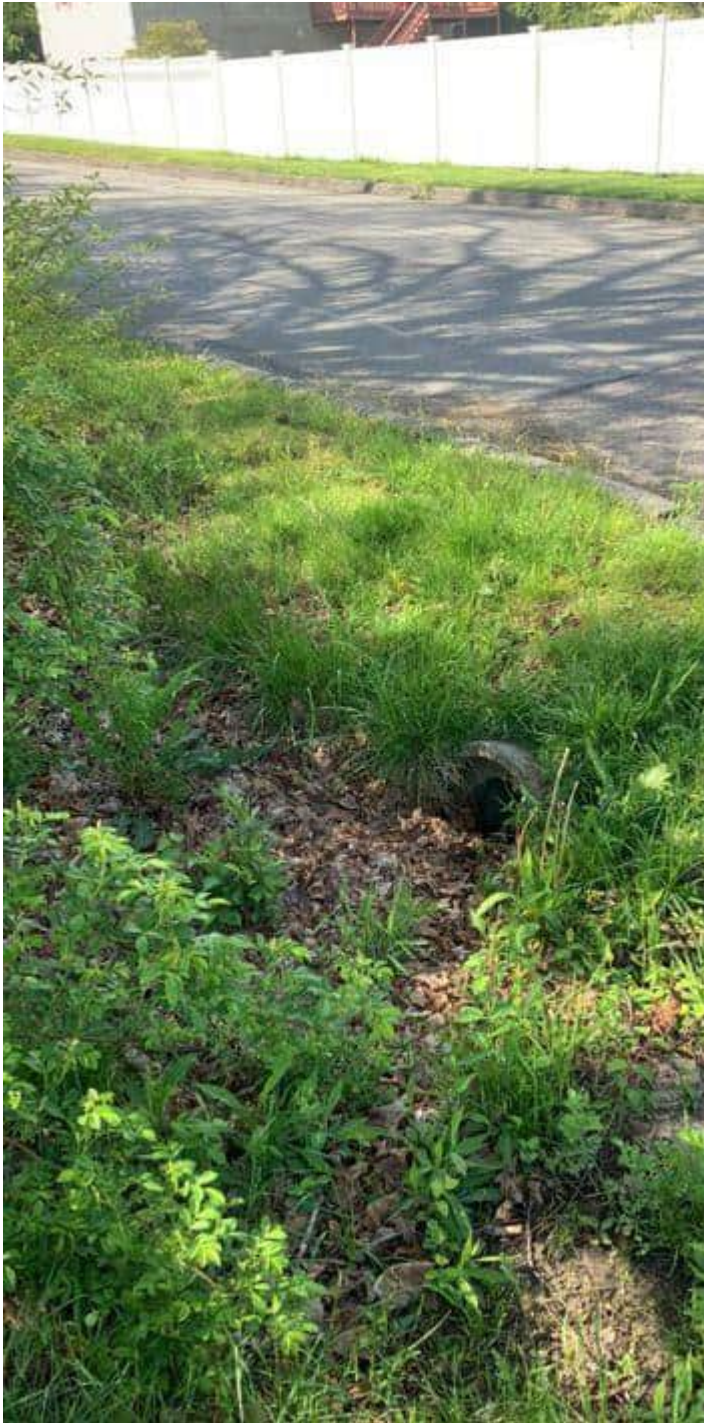
Infiltration trench outlet
