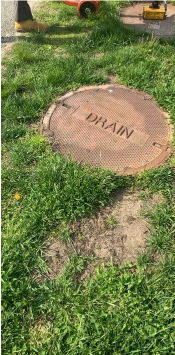
Outside second manhole
