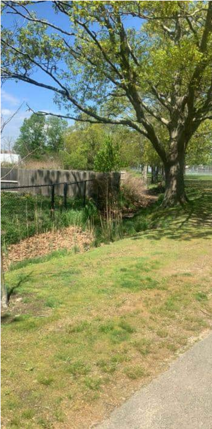
Section of swale leading to infiltration basin
