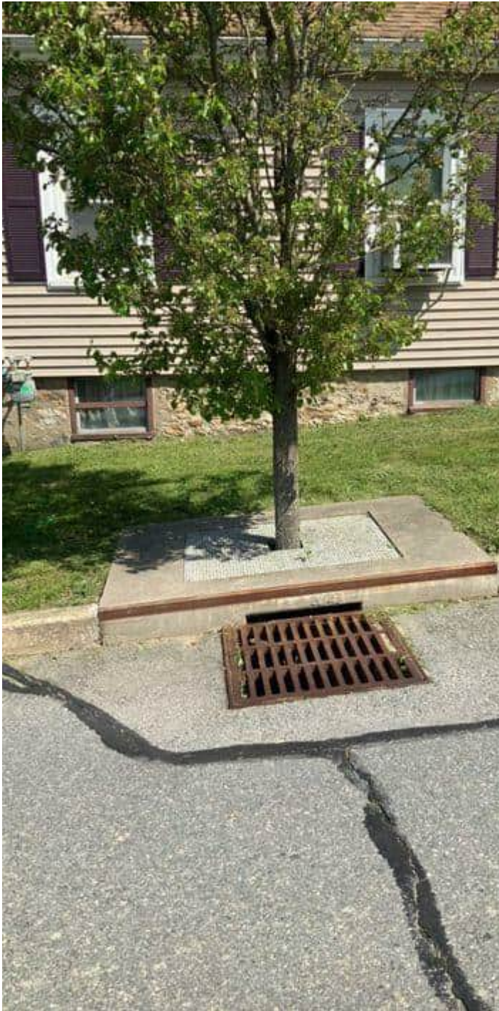
Outside tree box filter
