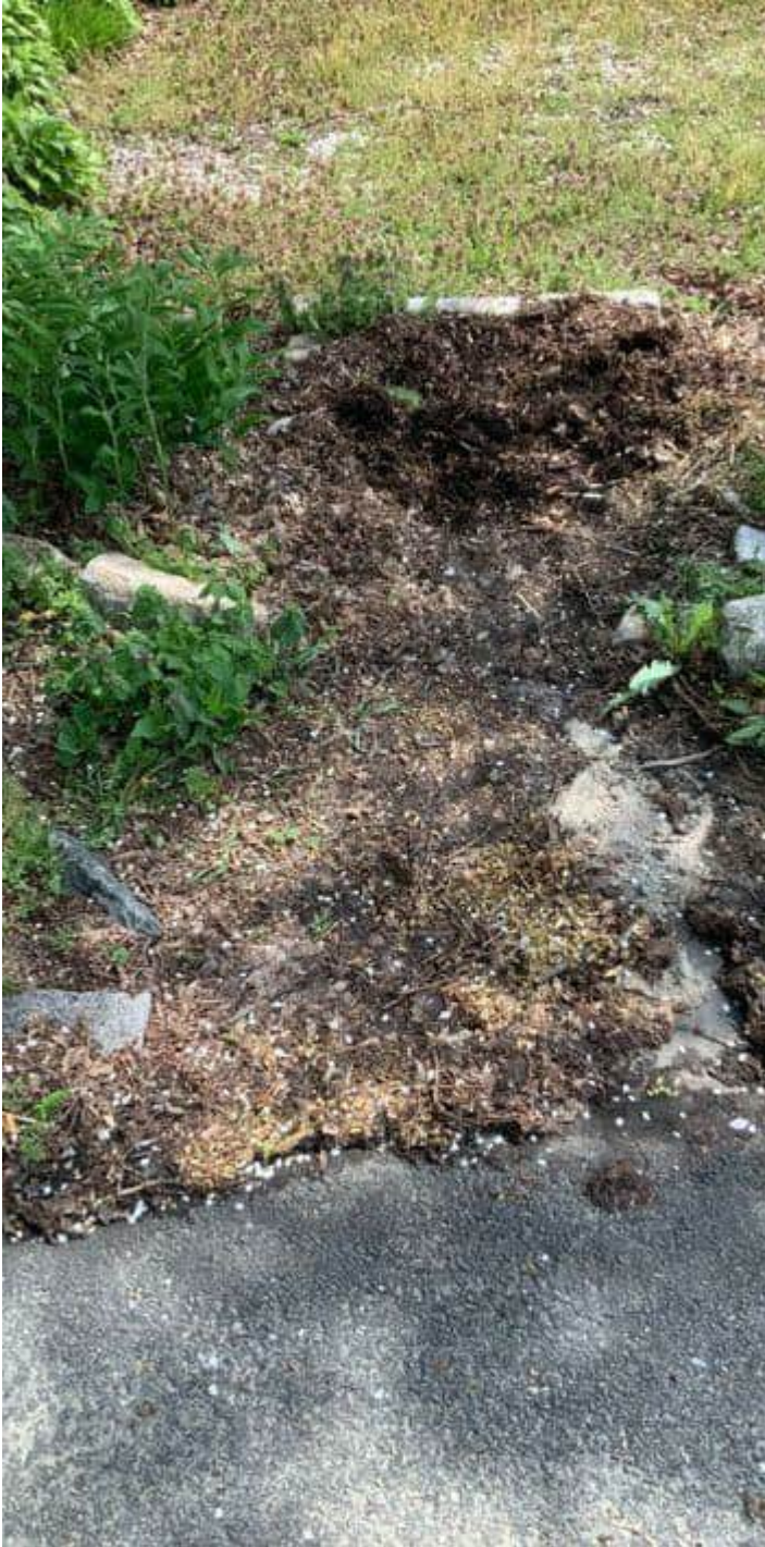
Clean Sediment and debris from inlet channel
