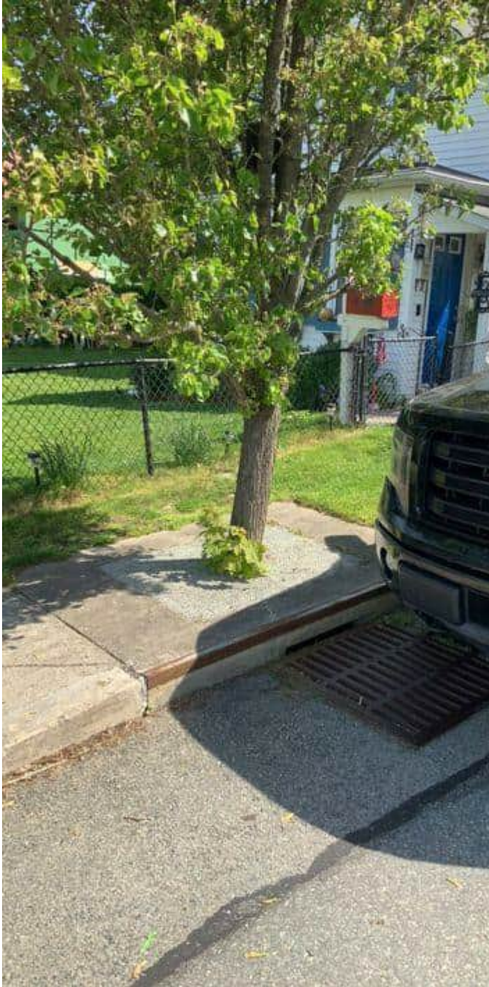
Outside tree box filter 2
