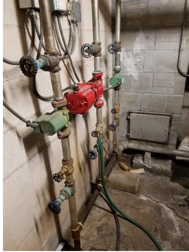
Fire Station – HW Zone Circulator Pumps
