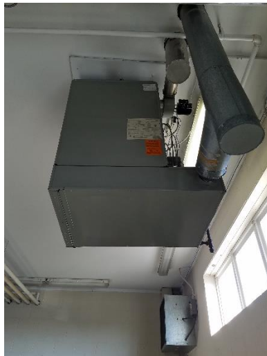
Police Station – Apparatus Bay Gas Fired Unit Heater
