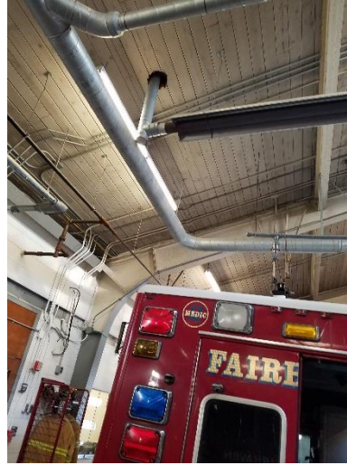
Fire Station – Gas Fired Radiant Heater
