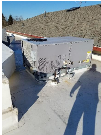
Police Station – Packaged Roof Mounted Air Handling Unit
