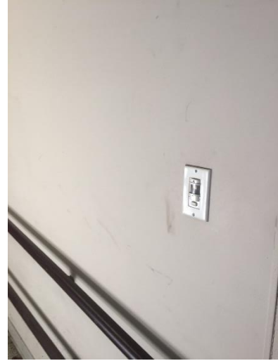
Typical OCC Sensor Switch
