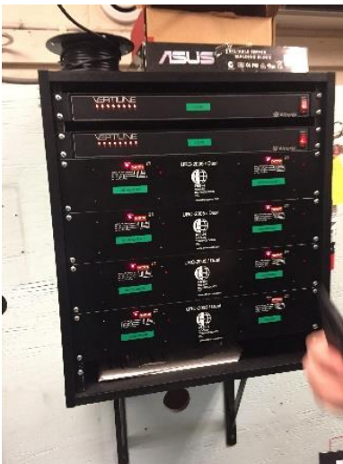
Access Control System Head End
