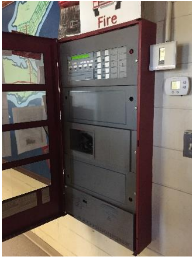
Fire Alarm Control Panel
