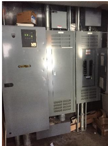
Transfer Switch and Emergency Distribution Panel
