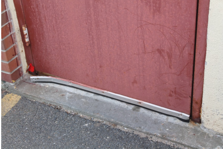
Photo 5: Damaged sweep at exterior door
