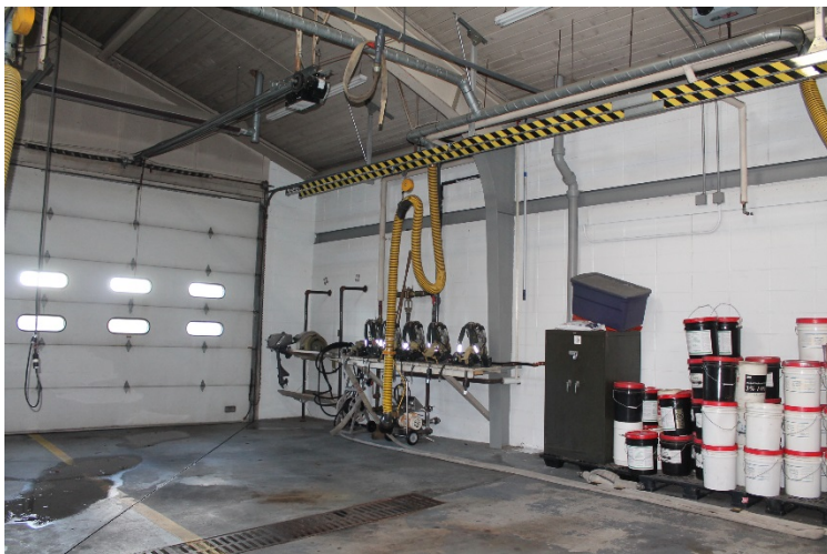
Photo 13: Ponding and peeling paint at apparatus bay floor
