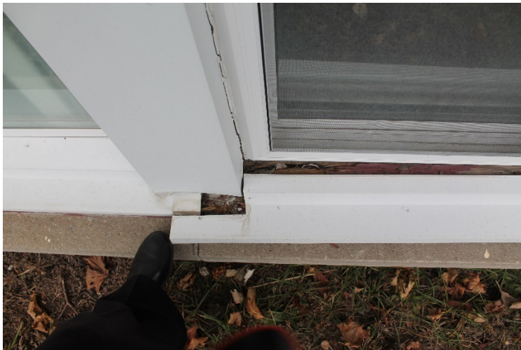
Photo 10: Wood sill is rotten below detached metal cap
