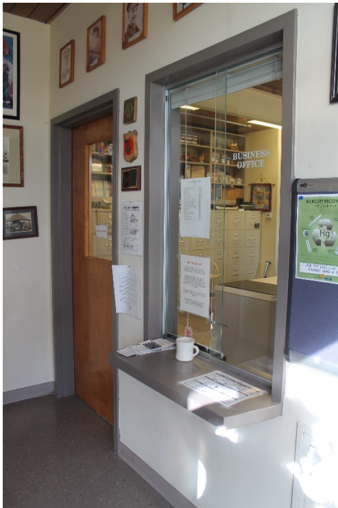
Photo 15: Transaction counters in fire station project into the accessible pathway
