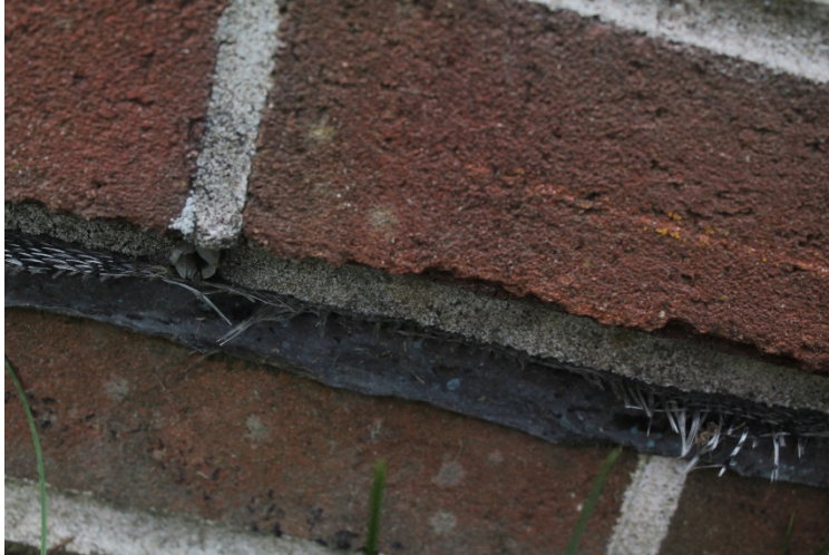
Photo 1: Deteriorated fabric flashing at wall base
