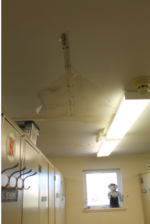
Photo 14: Water damaged gypsum wallboard ceiling in locker room
