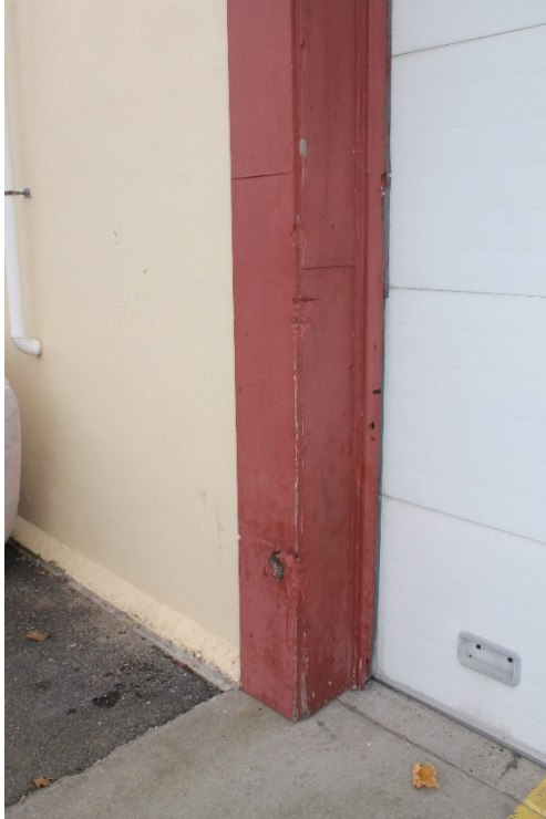
Photo 3: Rotten wood trim at overhead door
