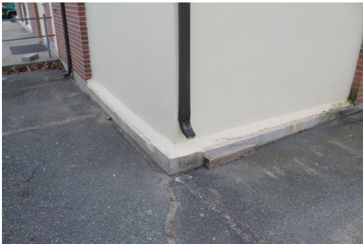
Photo 8: Downspout empties at low point where water drains back to building
