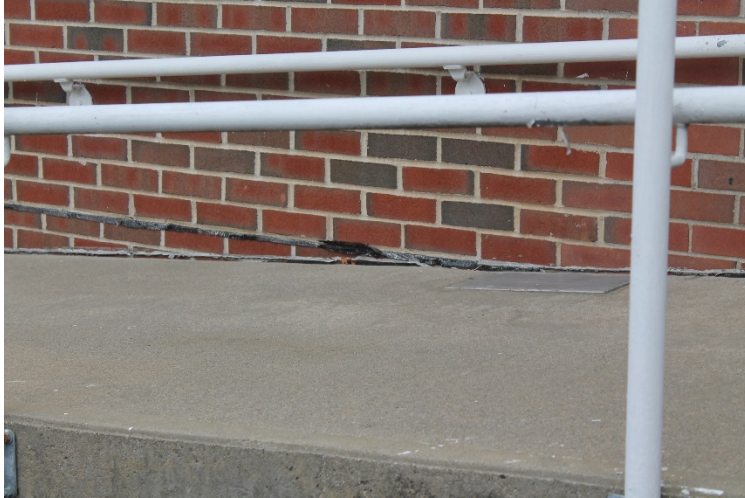
Photo 11: Flashing is not stepped at ramp, but dies into walking surface
