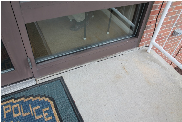
Photo 12: Joint where ramp/stair meets the building is deteriorated and open
