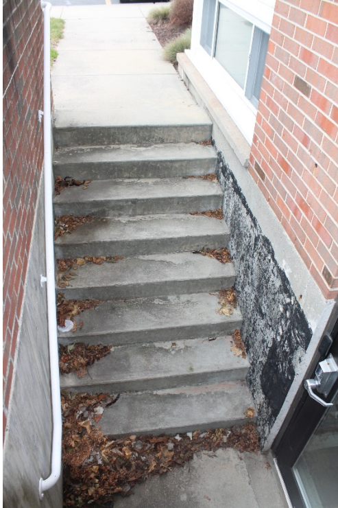
Photo 9: Exposed waterproofing in areaway
