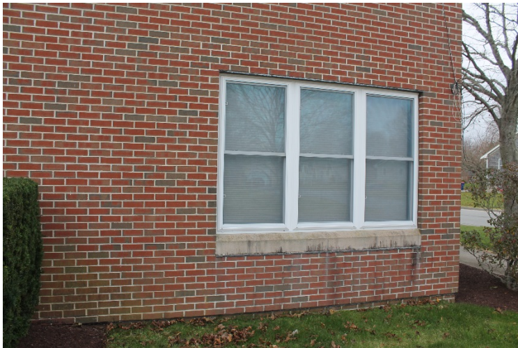
Photo 2: Deteriorated fabric flashing at window head, precast sill and base of wall
