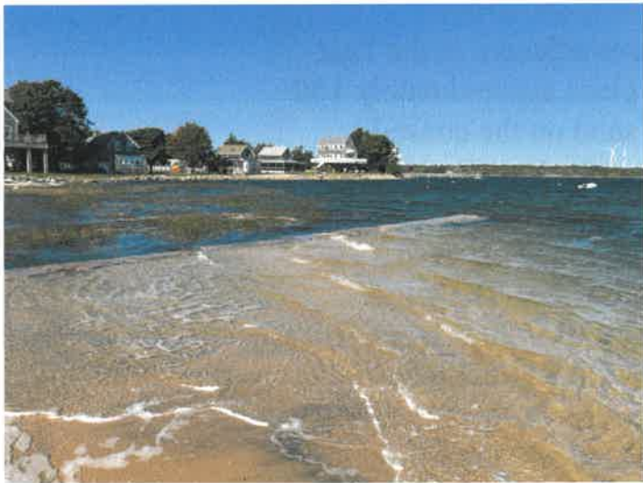
Photo 5 – West-end jetty during spring tide with north wind; overtopping visible.
