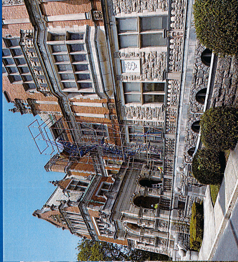
South Facade Repointing/Repair/Roof Replacement
