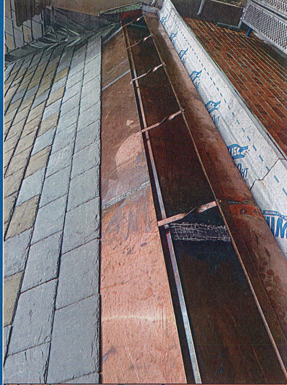
West Auditorium Gable Roof, Flashing, and Gutter Repair
