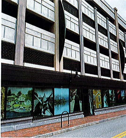
Figure 10. Security grills on a parking garage in Portsmouth NH are designed to provide an additional level of visual interest to the façade. The lower story of this garage incorporates storefront windows featuring local art. In the SMGOD, ground floor spaces adjacent to streets must be occupiable so this approach would not be acceptable.
