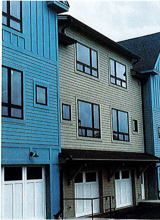
Figure 11. These townhouses in Northampton, MA have side-facing garage entrances accessed off a narrow driveway. The detailing of the garage doors and their surroundings is consistent with the rest of the building. (Dodson & Flinker)
