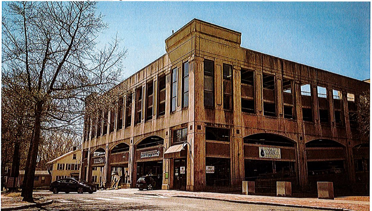
Figure 9. The design of a parking structure in Northampton MA reflects buildings in its area. The first and second parking levels are integrated into a set of what appear to be tall arched opening. Upper stories have well-proportioned openings. Concrete detailing on the building reflects elements of brick storefronts in the area.
