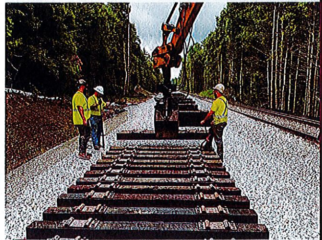
Setting ties on the right of way
