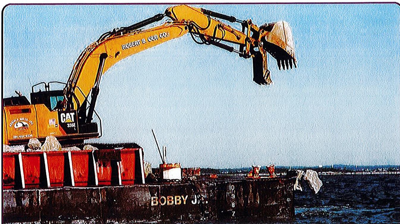
Claw dropping some SCR granite pieces into local waters to build up the reef
